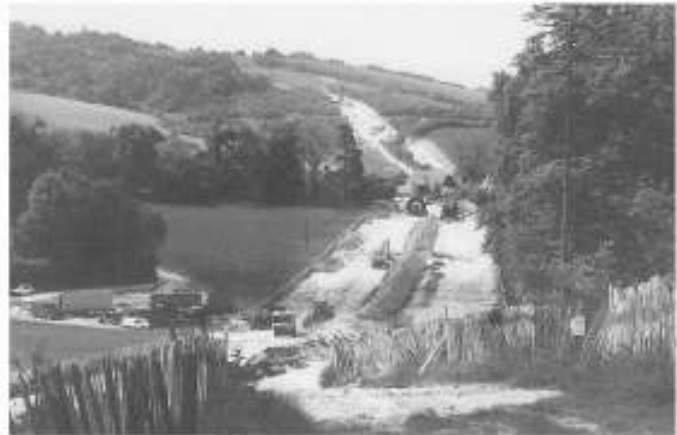
Image of "full undergrounding" from National Grid's current booklet "Overhead or Underground? National Grid's approach."
