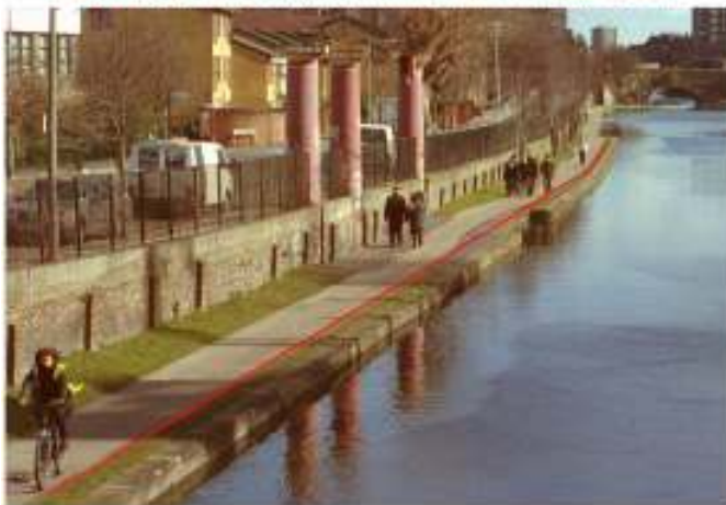
Above: Pylon and 400kV double circuit overhead transmission line seen from Dunford Bridge. Below: 'Undergrounding'/surface troughing (left of the red line) of a 400kV double circuit in the towpath of Regents Canal, London. Photographs 2006
