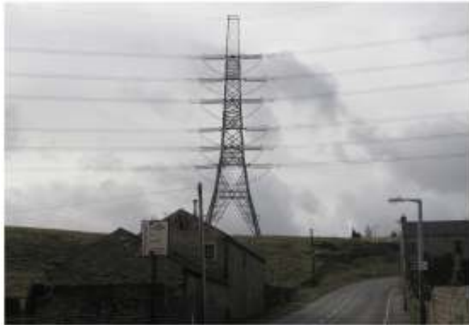
THESE TWO NG TRANSMISSION SYSTEMS CARRY THE SAME POWER
