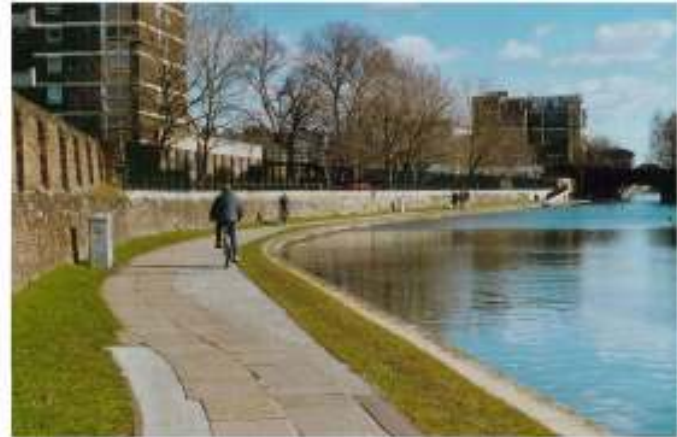
Pedestrian route above six 'undergrounded' NG 400kV cables in Regents Canal towpath, London. The track bed of the old Manchester to Sheffield railway appears to offer similar opportunities for 'undergrounding'
